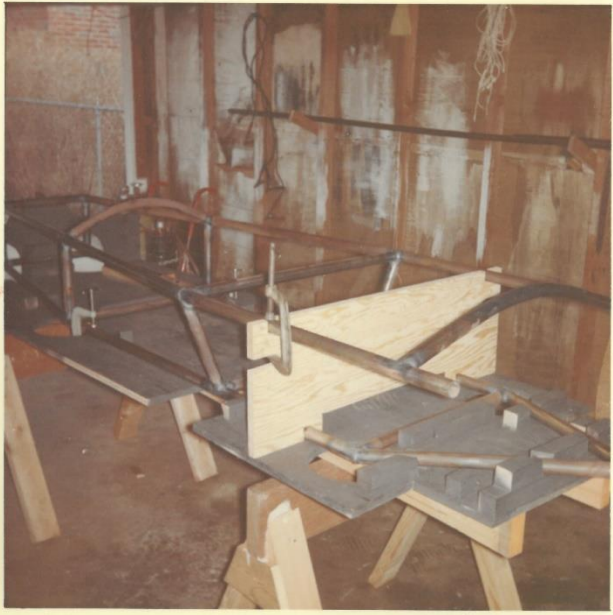
Frame Welded in Plywood Fixture
